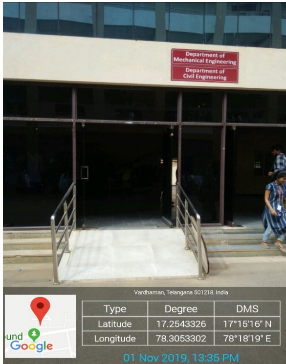
Block-2 Ramp and Hand Rails
