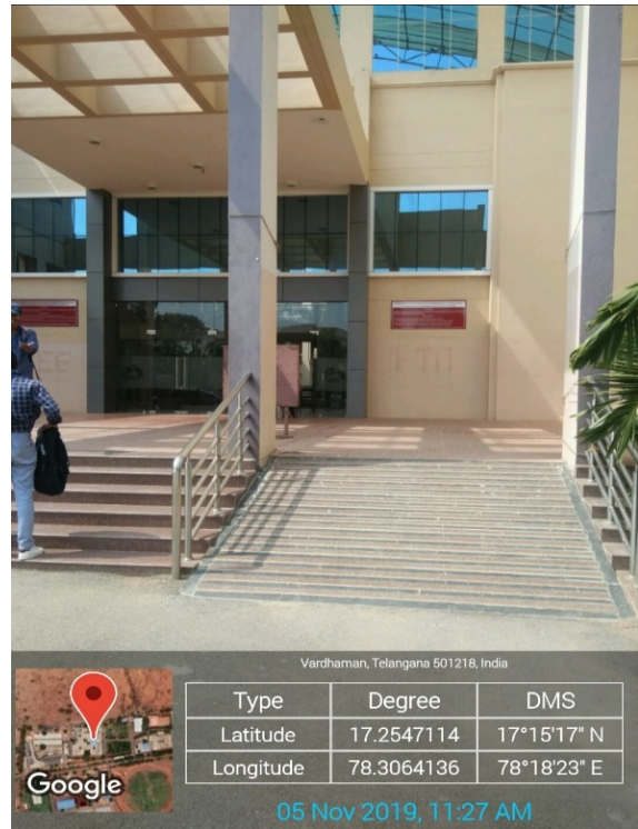
Block-3 Ramp and Hand Rails
